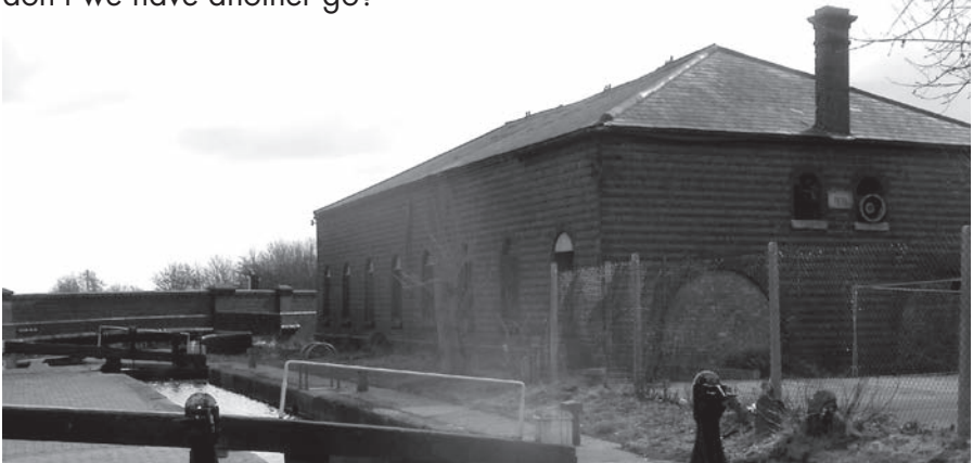
Gauging Station, Factory Locks, Tipton by Gavin Lawson
